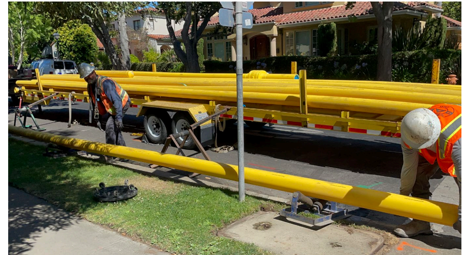
Installing new gas pipe for the Gas Main Replacement Project #24B
