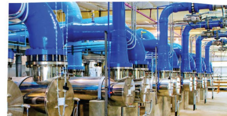
#3 UV LIGHT DISINFECTION AND ADVANCED OXIDATION
