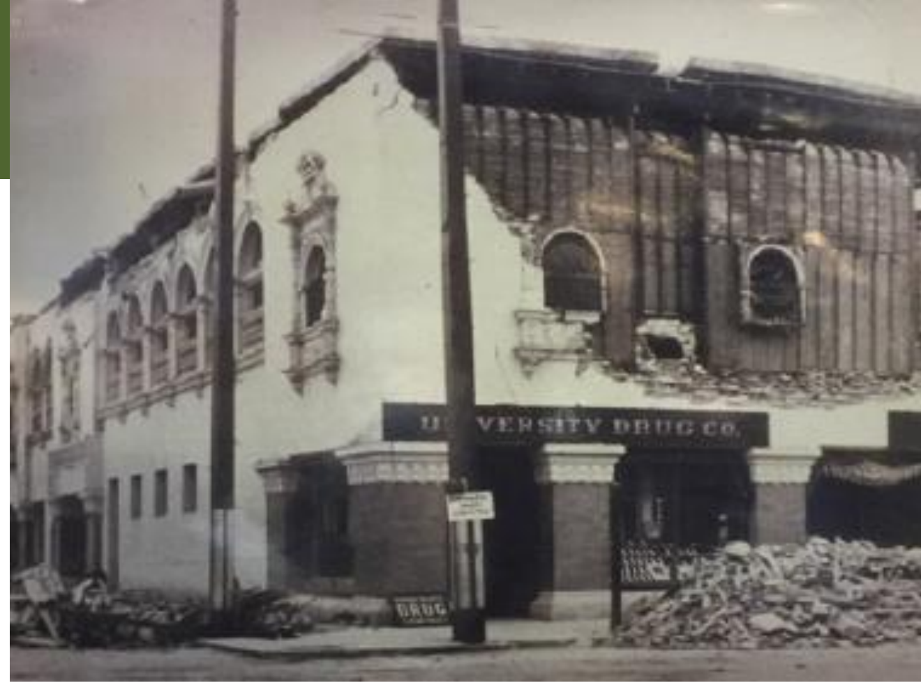
Image: Category I, Unreinforced Masonry Building Earthquake Damage
