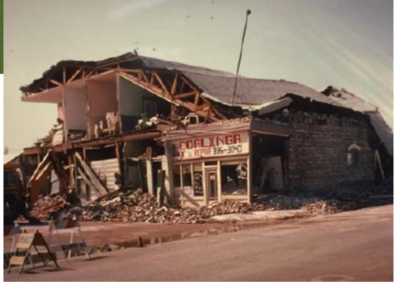
Image: Category I, Unreinforced Masonry Building Earthquake Damage
