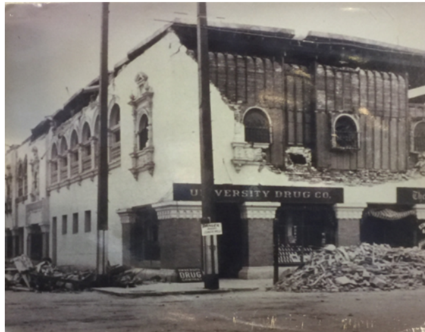
Figure 2: Category I, Unreinforced Masonry Building Earthquake Damage
