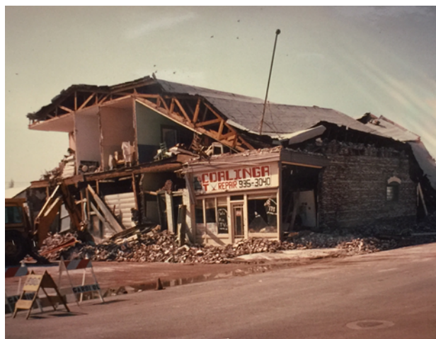
Figure 3: Category I, Unreinforced Masonry Building Earthquake Damage
